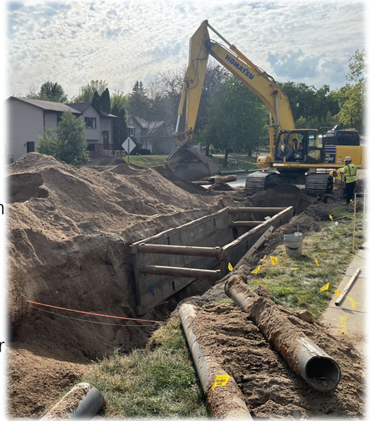
Water main replacement Cope Avenue (2022)
