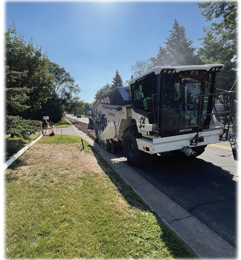
Reclamation on Cope Avenue (2022)
